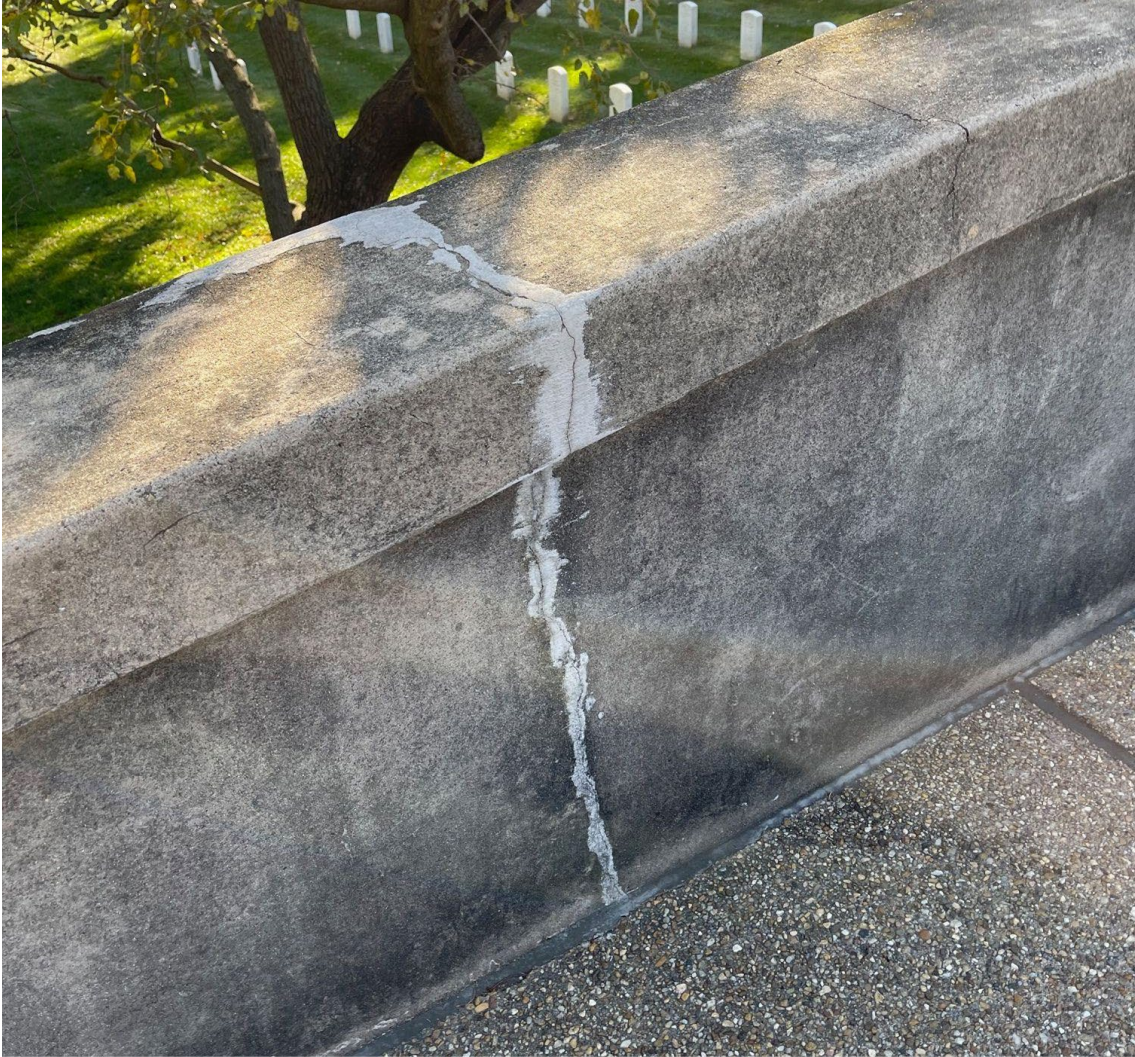
Details of cracking near the center of the East and West parapet walls
