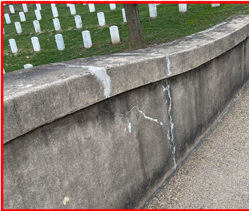
Detail of crack on the inside of the East parapet wall on Crook Walk bridge, before structural investigation
