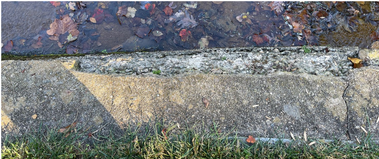
Detail image of cracking and concrete surface loss in the channel
