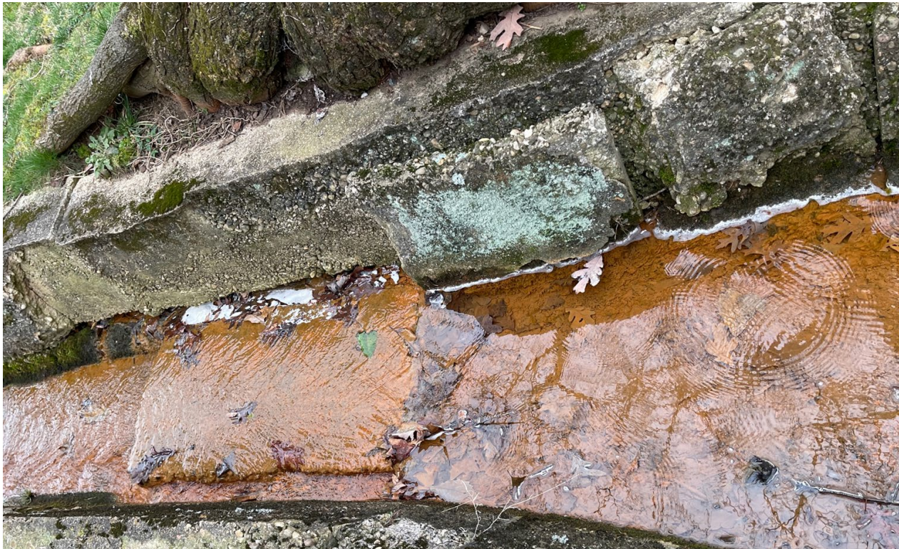
Detail photos of loose, deteriorated concrete panels in the Section 37 channel
