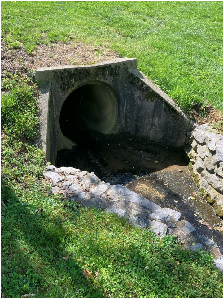
Culvert with granite sidewalls near Roosevelt Drive
