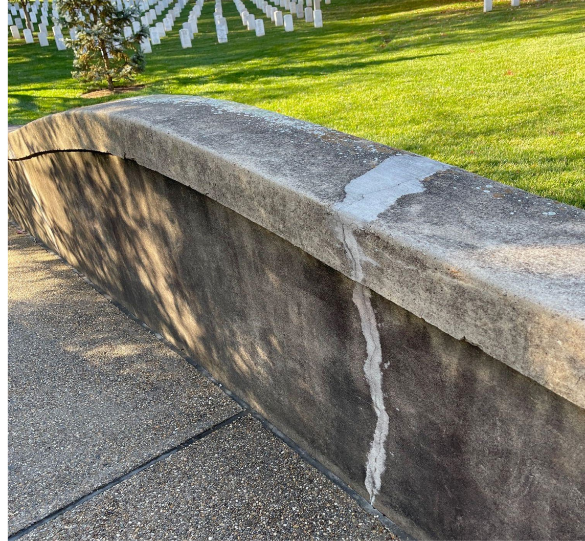
Details of cracking near the center of the East and West parapet walls
