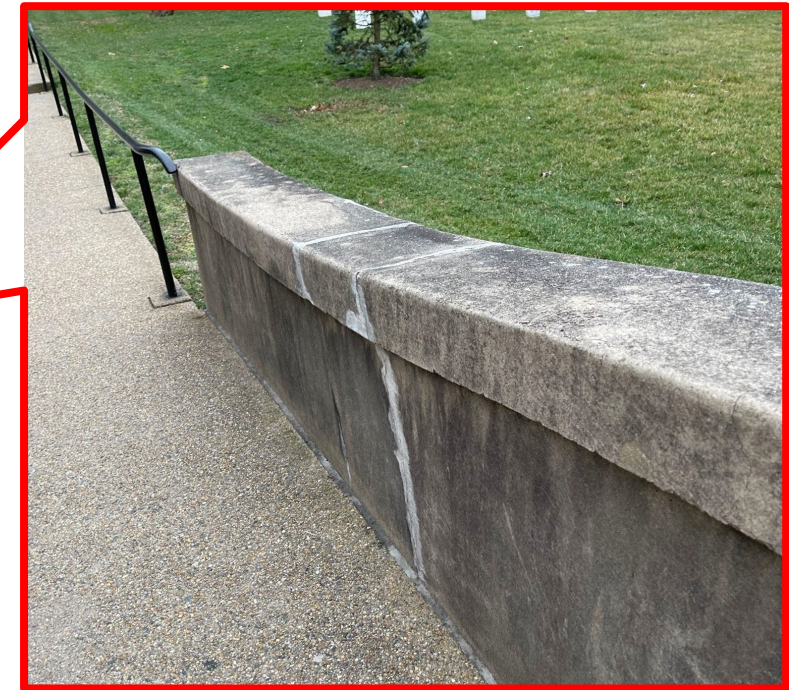
Detail of crack on the inside of the West parapet wall on Crook Walk bridge, before structural investigation
