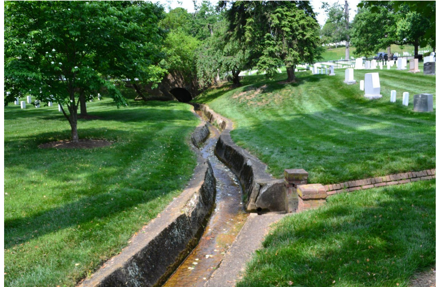
Section 37 drainage system, looking west toward the Crook Walk bridge, where the brick-lined channel connects with the concrete channel
