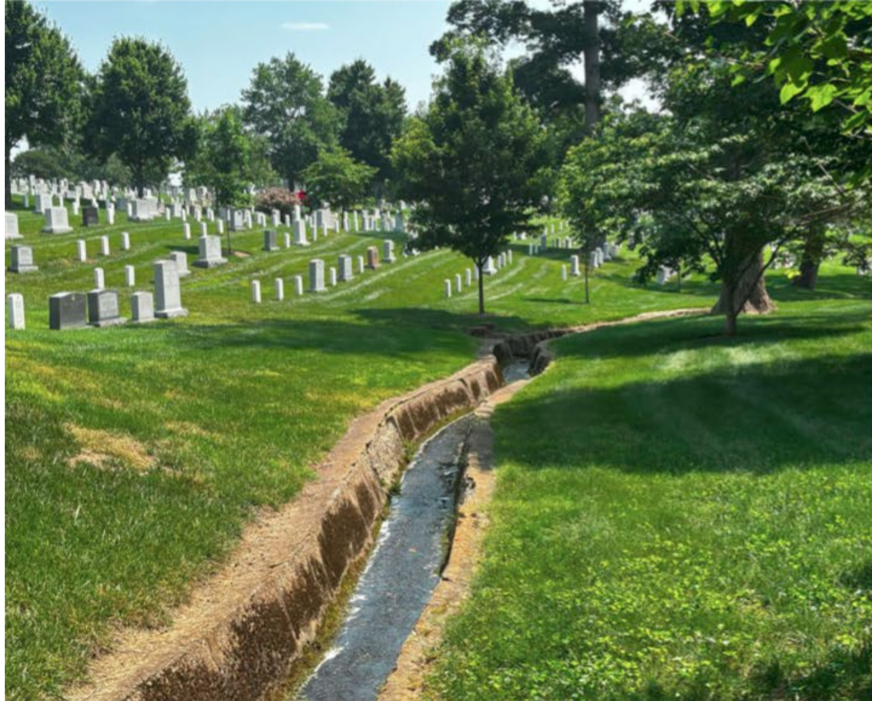
Existing Section 37 channel conditions, before rehabilitation
