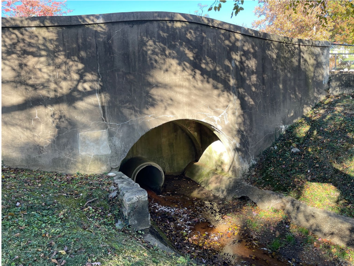
Eastern parapet wall, wingwalls, and culvert at Crook Walk bridge
