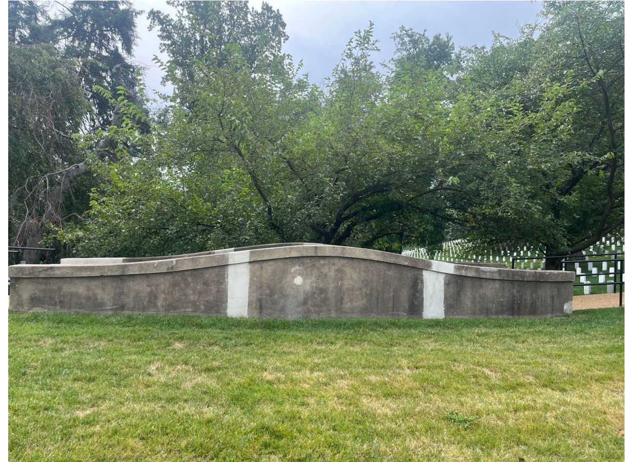
Western parapet wall of Crook Walk bridge, after structural investigation and temporary patching of cementitious parging and structural cracks
