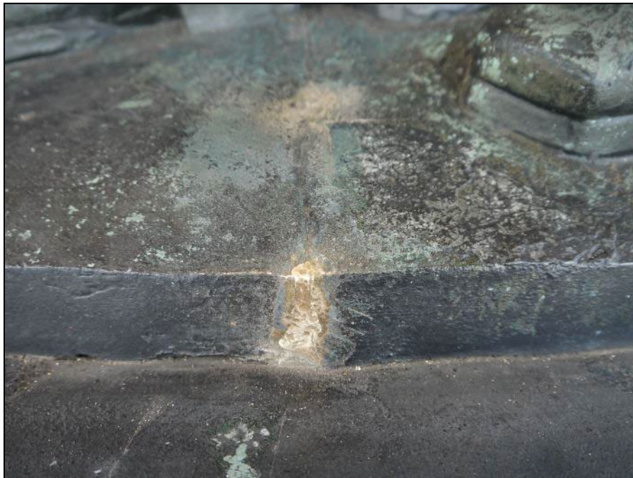
Figure 7. Bronze sheet peened in place to fill gap, part of the 2015 conservation treatment. Conservation Solutions, Inc., 2015.
