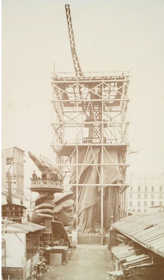
Figure 3. Photograph by Albert Fernique showing the steel internal bracing system in the Statue of Liberty, 1883.
