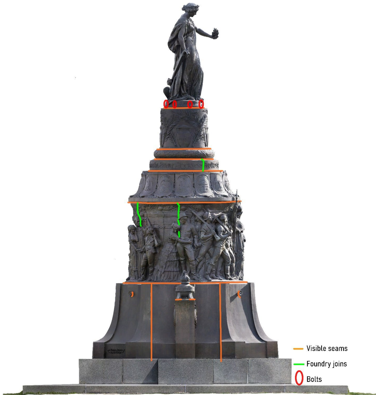
Figure 12. Confederate Memorial (000-1235), west elevation. Ortho-imagery generated from photogrammetric model from HABS 2022 Study. Image annotated to show visible seams made in the assembly of the monument at ANC, joins likely made at the Berlin foundry, and bolts which hold the top statue to the pedestal.
