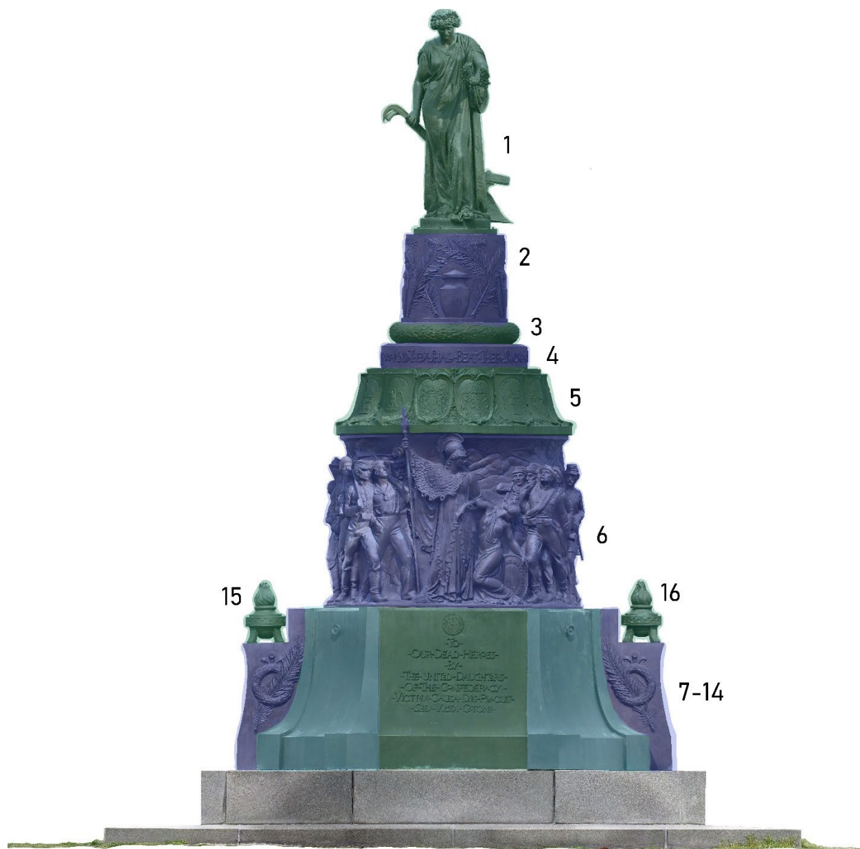
Figure 16. Confederate Memorial (000-1235), South elevation. Ortho-imagery generated from photogrammetric model from HABS 2022 Study. Image annotated to show major components of the monument and differentiate between bronze components.
