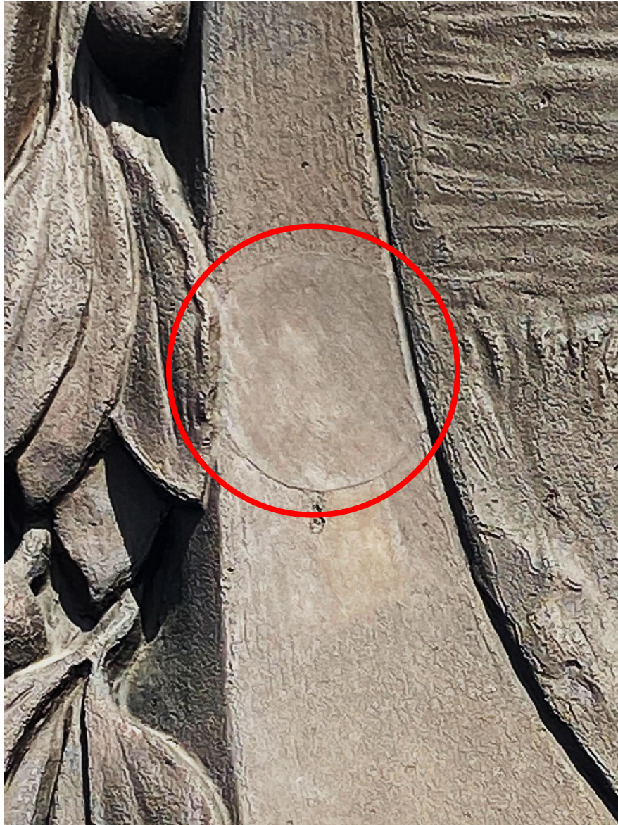
Figure 10. Possible attachment location for internal structural support. U.S. Army photo, July 14, 2023.
