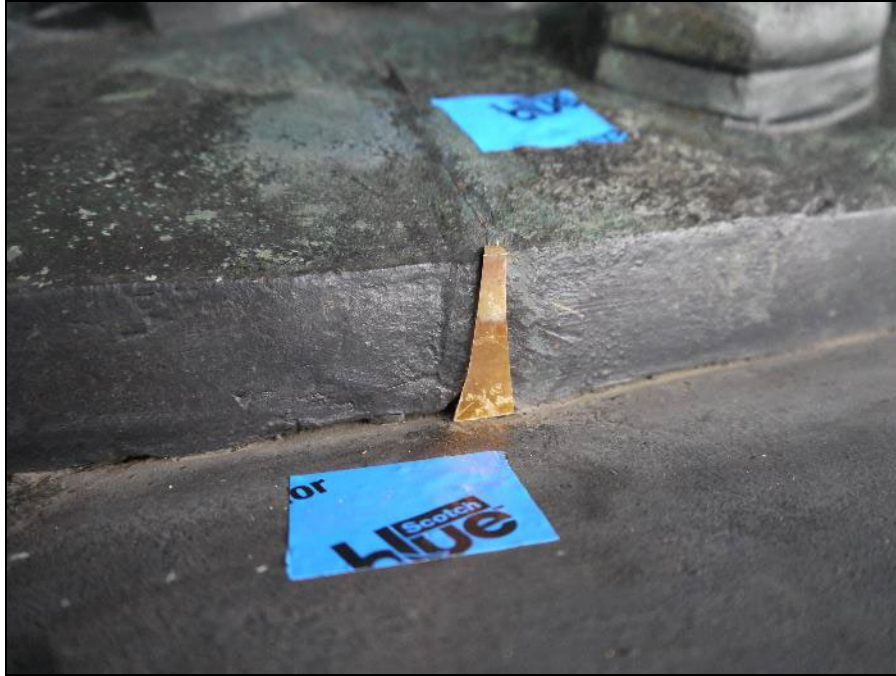
Figure 6. Bronze sheet installed to fill gap, part of the 2015 conservation treatment. Conservation Solutions, Inc., 2015.
