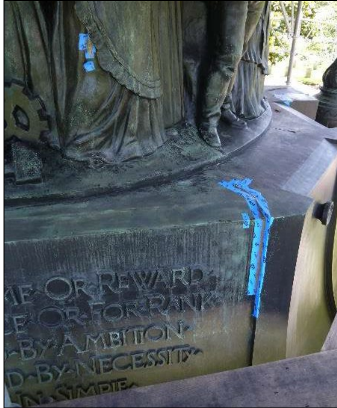
Figures 8–9. Installation of bronze-filled epoxy into open seam (during repair above, and after repair below) as part of the 2015 conservation treatment. Conservation Solutions, Inc., 2015.
