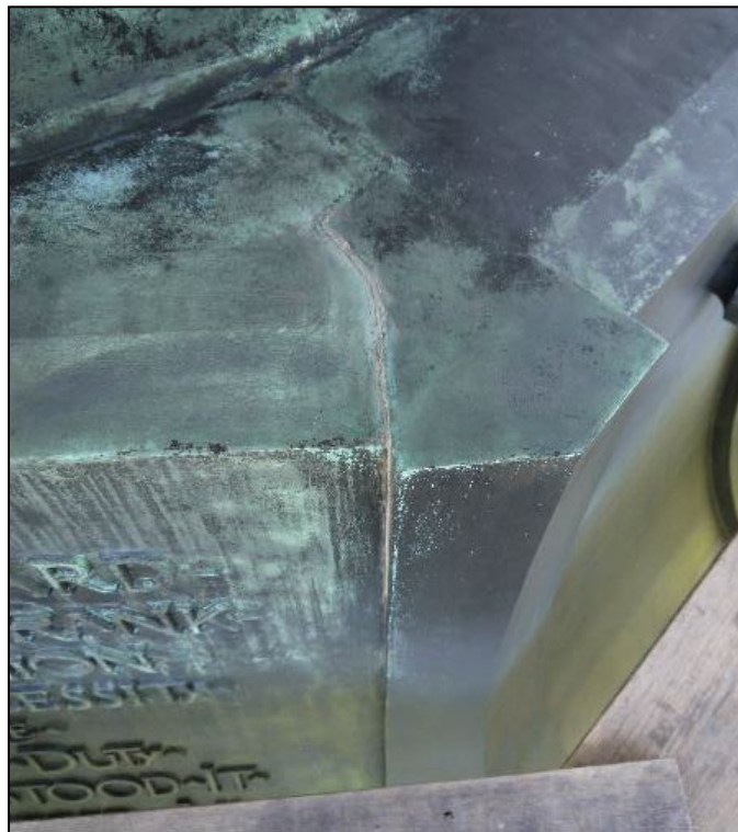
Figures 8–9. Installation of bronze-filled epoxy into open seam (during repair above, and after repair below) as part of the 2015 conservation treatment. Conservation Solutions, Inc., 2015.
