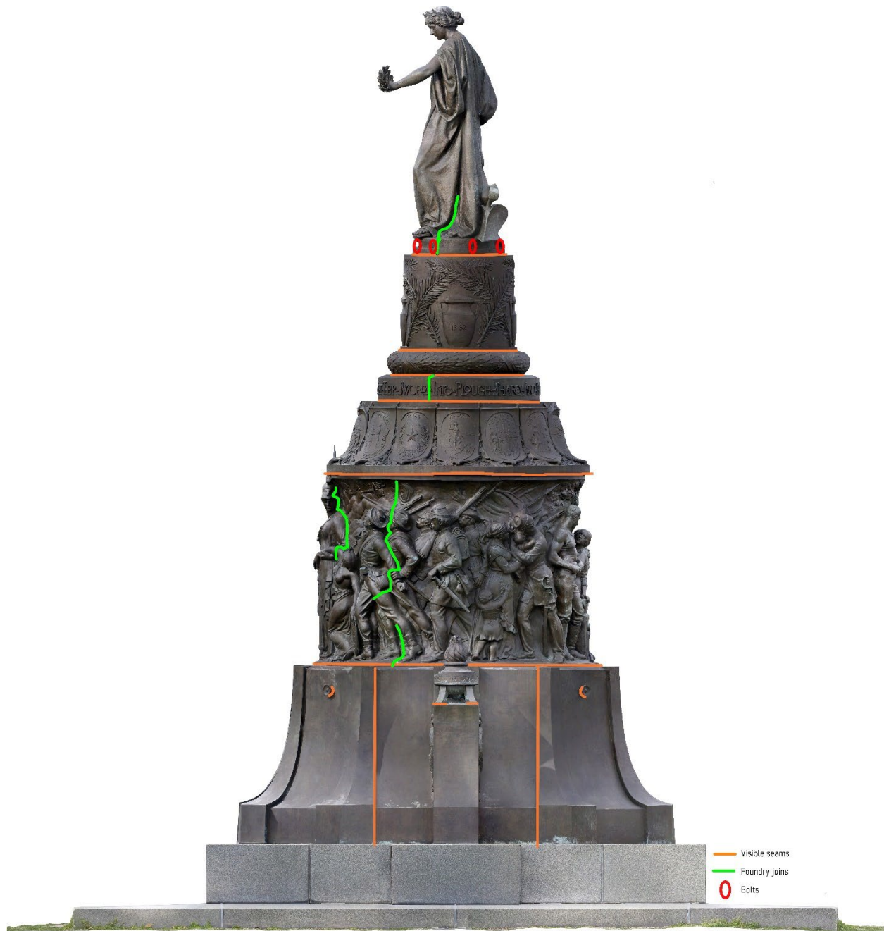
Figure 14. Confederate Memorial (000-1235), east elevation. Ortho-imagery generated from photogrammetric model from HABS 2022 Study. Image annotated to show visible seams made in the assembly of the monument at ANC, joins likely made at the Berlin foundry, and bolts which hold the top statue to the pedestal.
