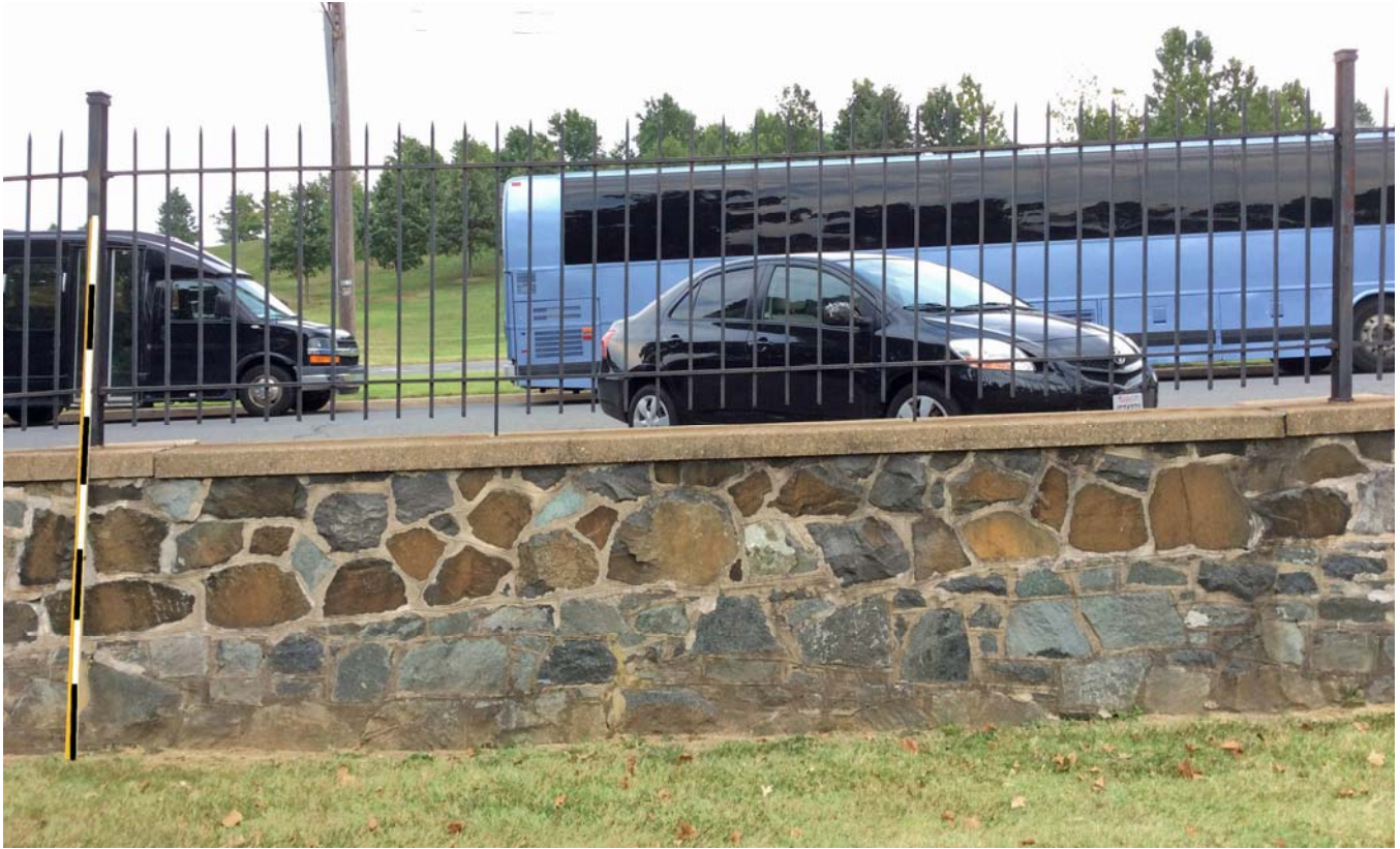
Figure 19- Boundary wall acting as a retaining wall
