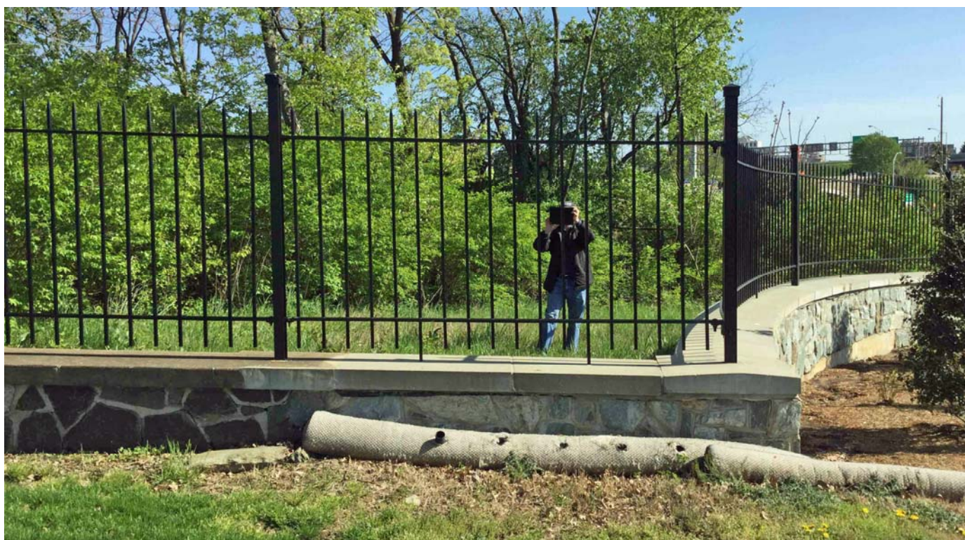
Figure 31- Wall Transition #2 at the east end of the study area
