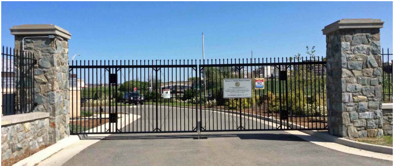
Figure 29- Secondary service area gate serving a parking area
