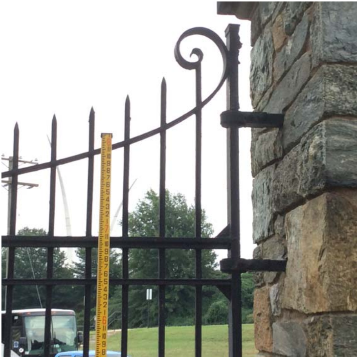
Figure 11- Detail of South/Clayton Gate
