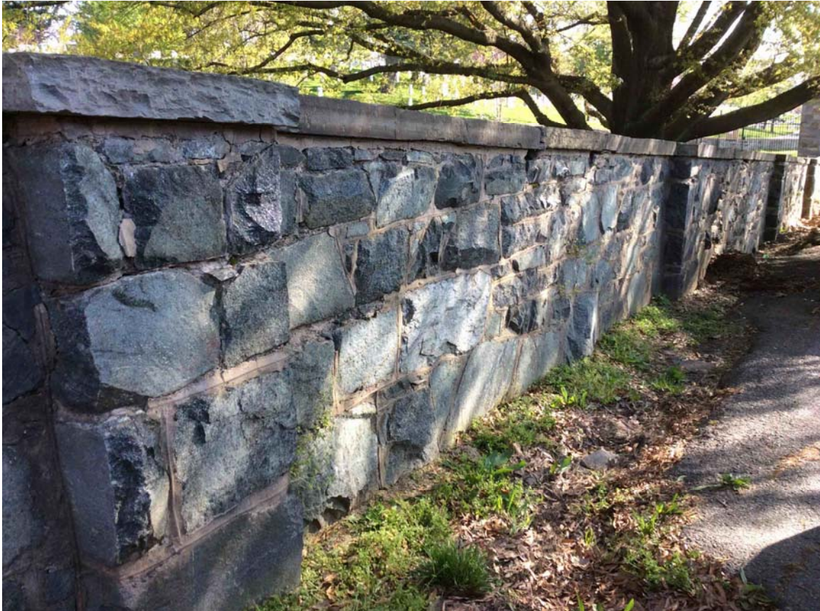
Figure 7- Westernmost section of boundary wall in study area
