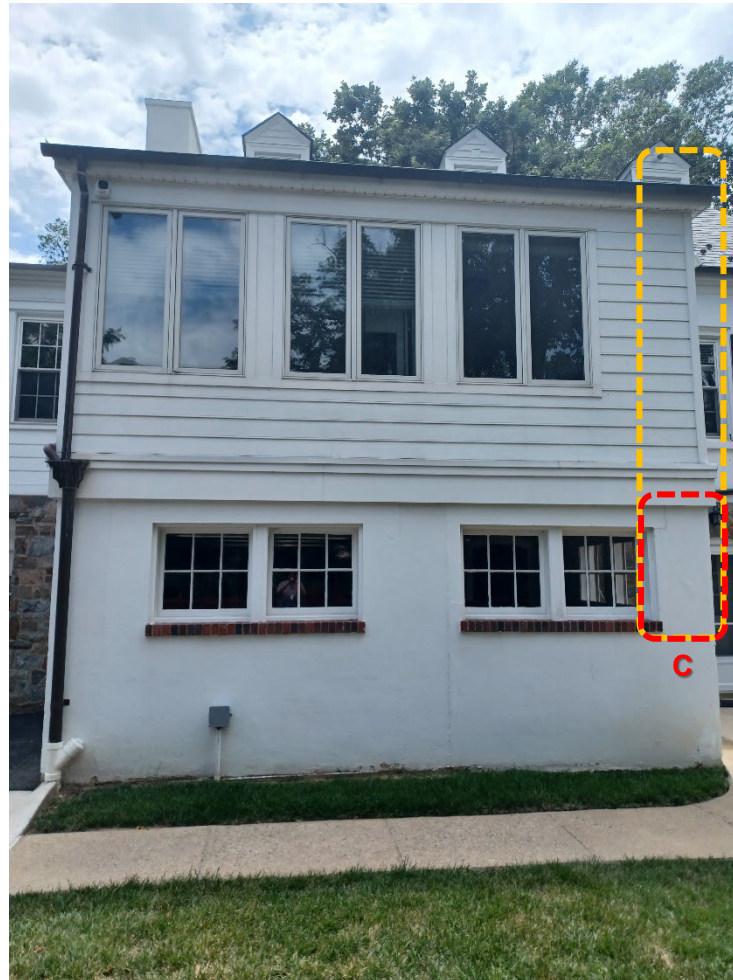
Superintendent's Lodge #1: Rear addition & garage looking northwest (left), southwest (center), and southeast (right). Shows elevations where fan/ventilation pipe may be located. The proposed ventilation system will penetrate through the garage wall. The proposed locations for the penetration are outlined in red . The proposed locations for the copper pipe to extend up the facade are outlined in yellow . The copper ventilation pipe must extend above the roofline. (U.S. Army photos by Jeremy Jordan / ANMC)
