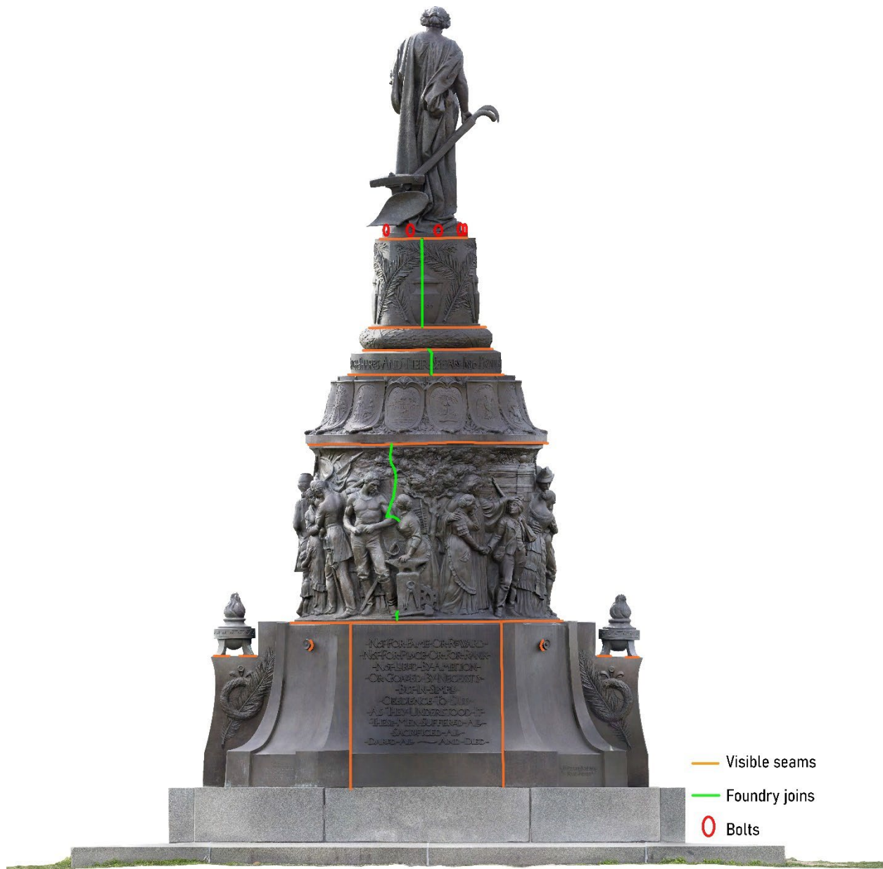
Figure 13. Confederate Memorial (000-1235), north elevation. Ortho-imagery generated from photogrammetric model from HABS 2022 Study. Image annotated to show visible seams made in the assembly of the monument at ANC, joins made at the Berlin foundry, and bolts which hold the top statue to the pedestal.
