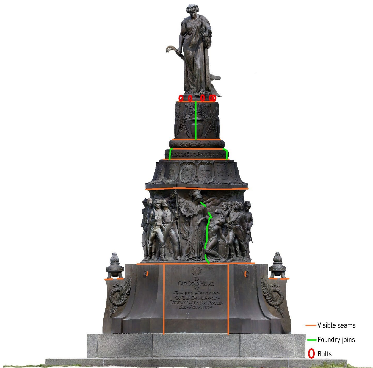
Figure 11. Confederate Memorial (000-1235), south elevation. Ortho-imagery generated from photogrammetric model from HABS 2022 Study. Image annotated to show visible seams made in the assembly of the monument at ANC, joins likely made at the Berlin foundry, and bolts which hold the top statue of the South to the pedestal depicting the four cinerary urns.
