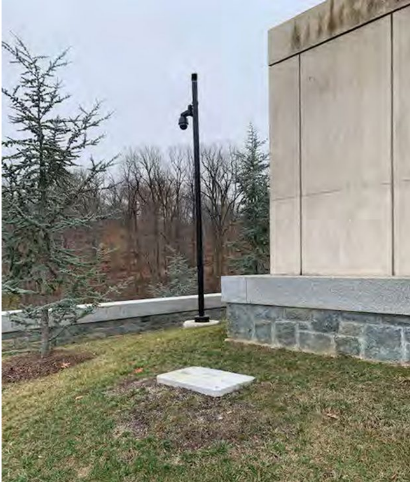
1 Illustration of the proposed combined Wi-Fi and CCTV camera pole looking Southeast. The pole is two feet taller than the existing pole to achieve proper distribution of coverage. Omni 1 Wi-Fi/CCTV Pole located at the far East Corner of the Millennium Columbarium off of Lewis Drive.
