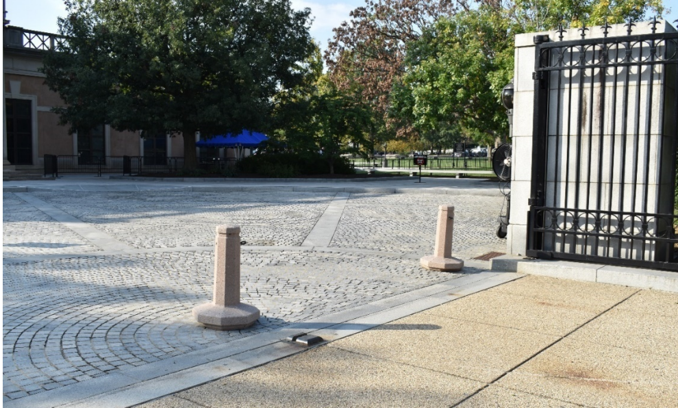
10 11 Figure 2-11. Welcome Center Concrete Bollards
