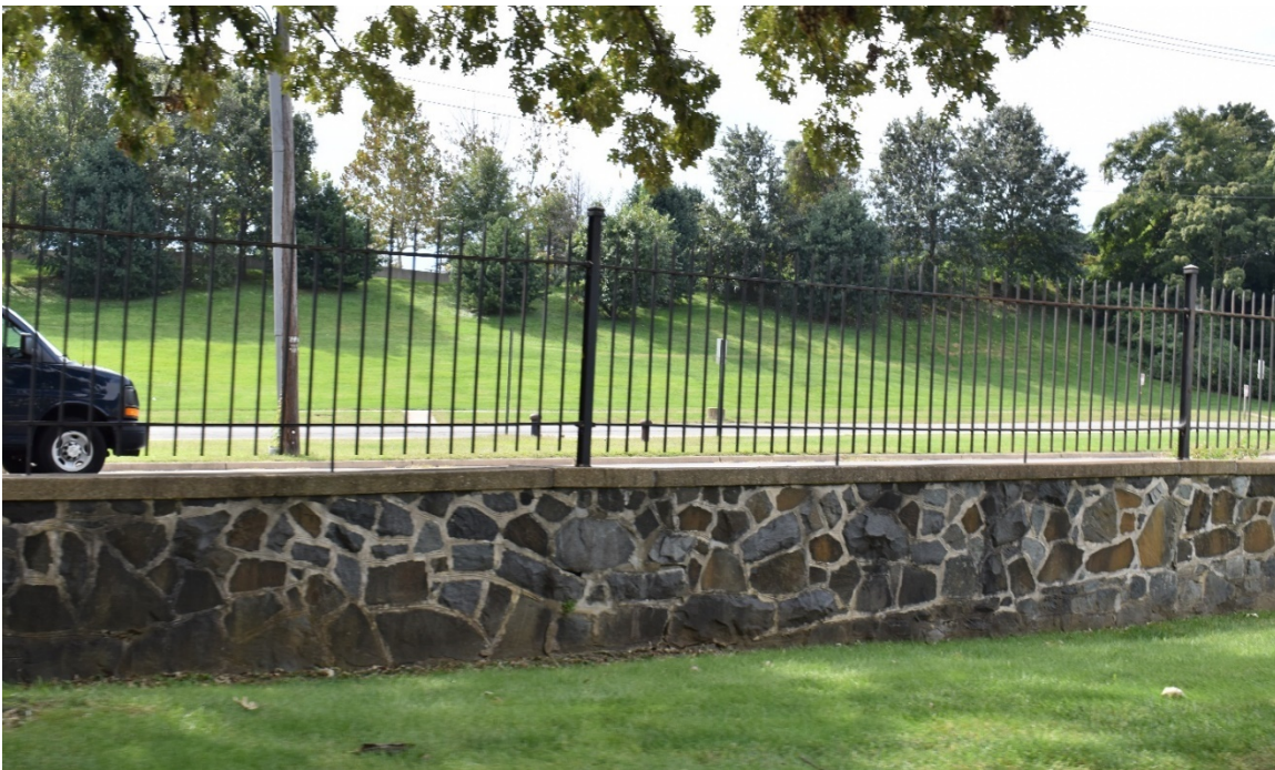
Figure 2-14. Example of Masonry Wall with Steel Fence Topper
