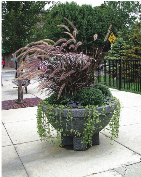
12 13 Figure 2-12. Example Concrete Planter Barrier
