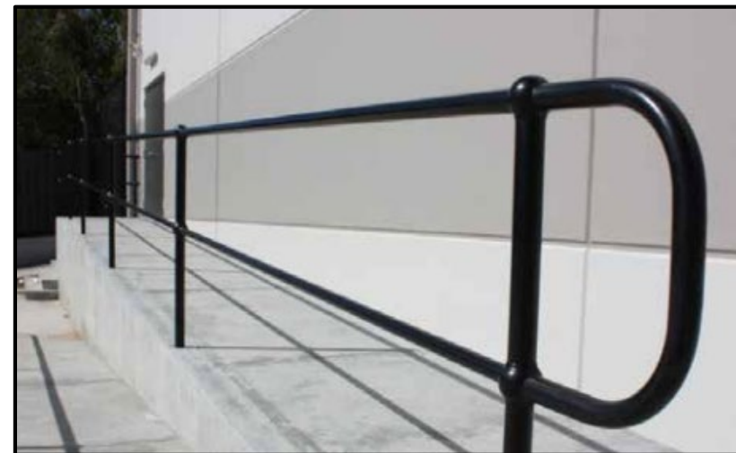
Proposed replacement railing for Crook Walk - black steel pipe and ball design with the "knuckle" at the joints
