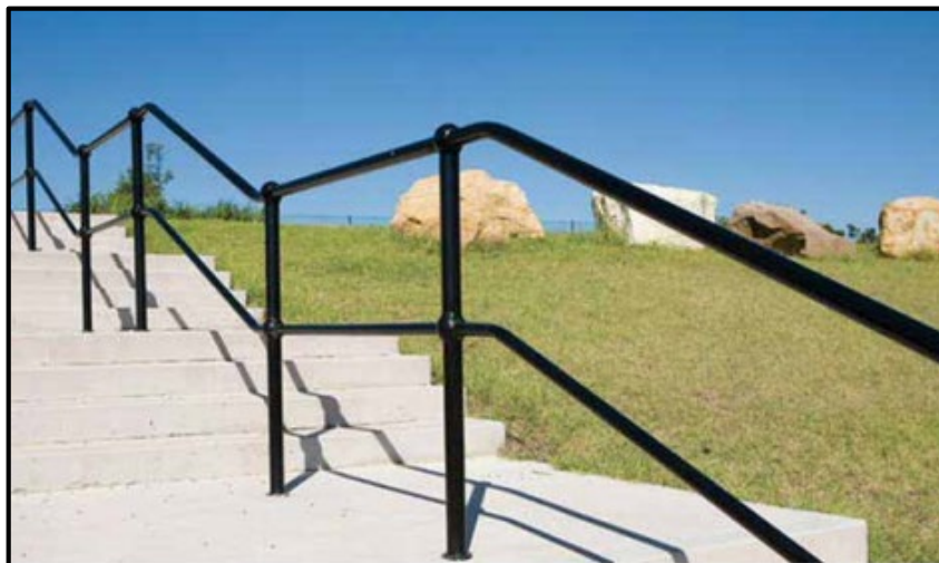
Proposed replacement railing for Crook Walk - black steel pipe and ball design with the "knuckle" at the joints
