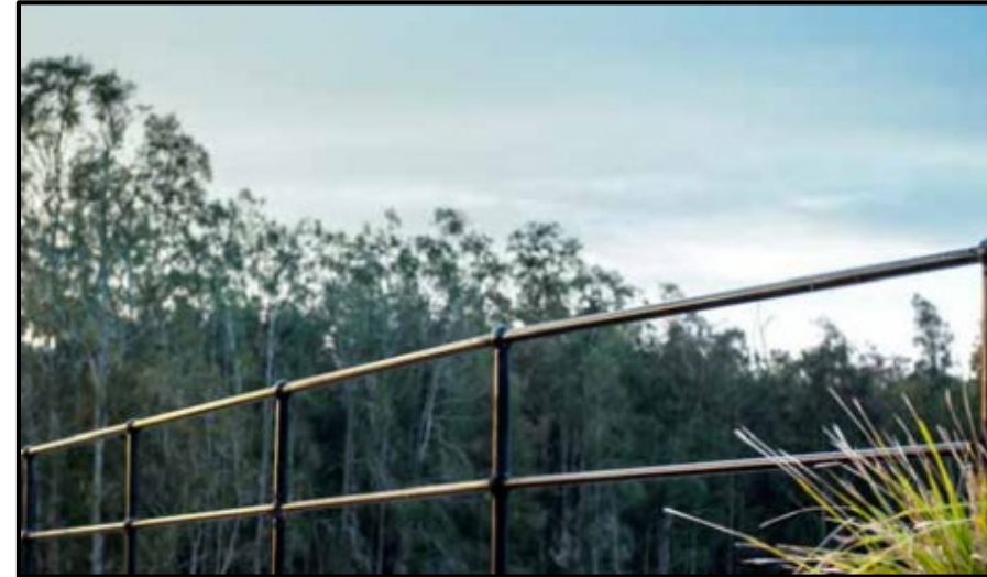
Proposed replacement railing for Crook Walk - black steel pipe and ball design with the "knuckle" at the joints
